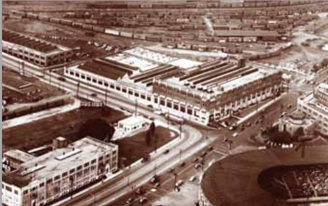
Loblaw Groceries Co. Limited Head Office & Warehouse.
